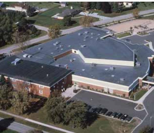
Versico Roofing Systems' EPDM membranes offer an optimal solution for nearly any low-slope roofing situation. EPDM is a durable material that has more than 50 years of proven, in-field performance. With significant physical property advantages, warming benefits in northern climates, and innovations in product technologies, EPDM is still defining the standard in the commercial roofing market. Below are the top 10 reasons to consider EPDM on your next roofing project.
